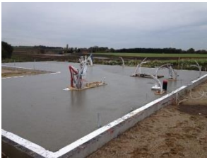
Phase 3a – fundament
