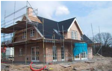
Phase 3c – roof
